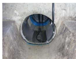
Installation of sensor in tube
